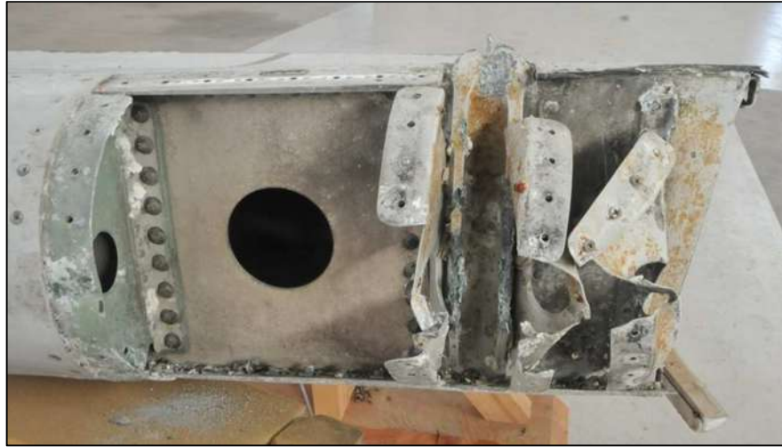
Planche 24 : Hinge fitting on the outboard side
